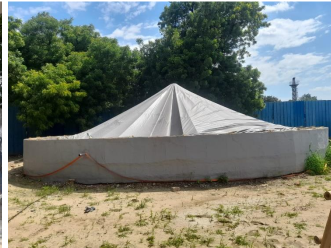
Bio digester under construction
