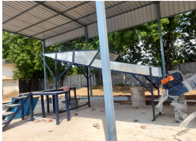
MRF under construction
